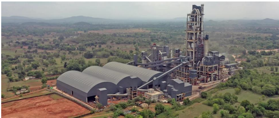
Shiva Cement Plant at Telighana, PO: Birangatoli, Tehsil- Kutra, District-Sundargarh, Odisha
